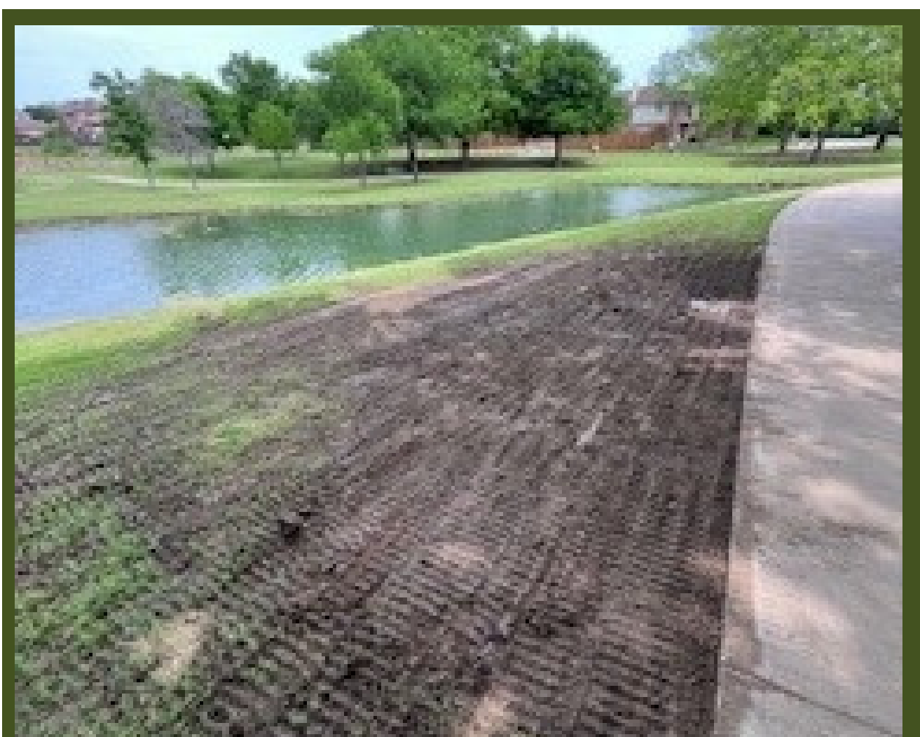
EMERALD BAY EROSION REPAIR
